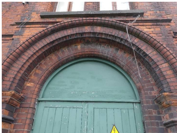
Gauged-brick arch-head with outer archivolt springing from pilasters
