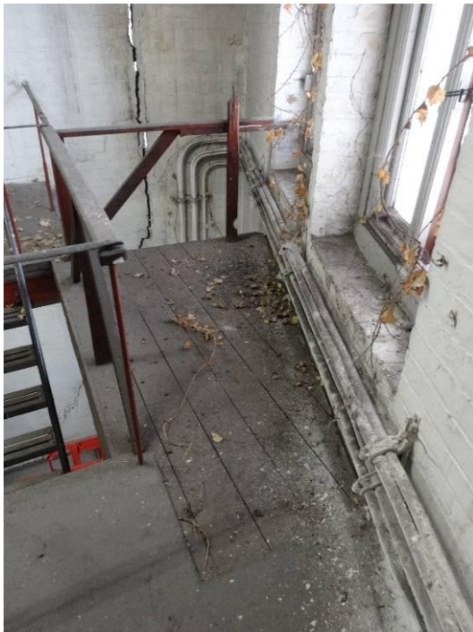
Eastern end of first-floor level. Timber floor adjacent to window
