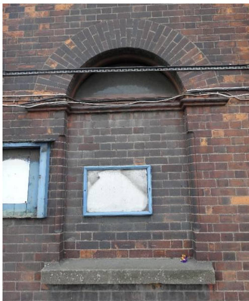
Blind round-arched opening on north elevation
