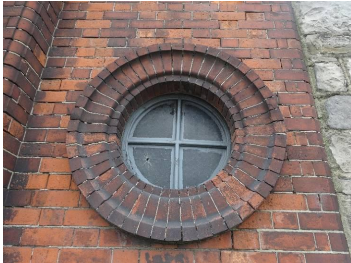
Gauged brick surround to circular window at ground-floor level
