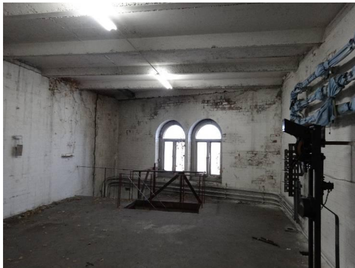
First-floor level of the ESB sub-station, looking west
