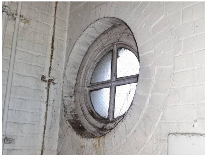
Circular window adjacent to entrance door
