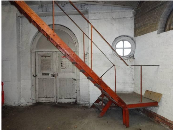
Steel stairs rising from ground floor to first-floor level
