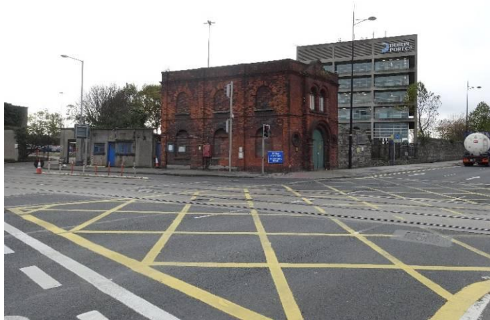
The corner-sited ESB sub-station at the junction of East Wall Road and Alexandra Road
