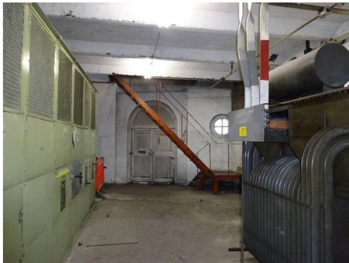
Ground-floor level of sub-station, looking west to entrance door
