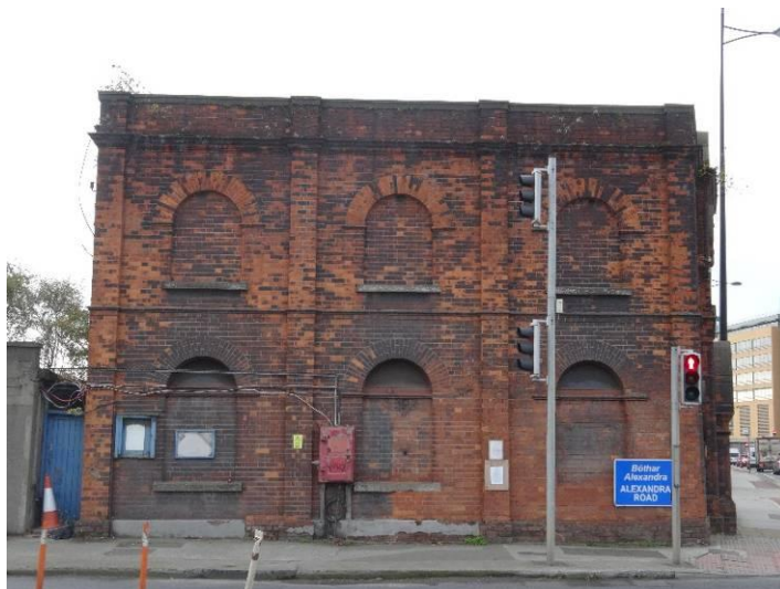
Three-bay, two-storey elevation to Alexandra Road
