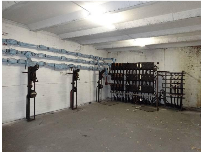
First-floor level of the ESB sub-station, looking east
